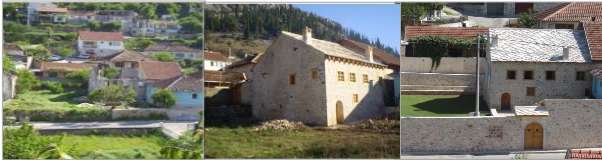
HIDR 1 before and after reconstruction
