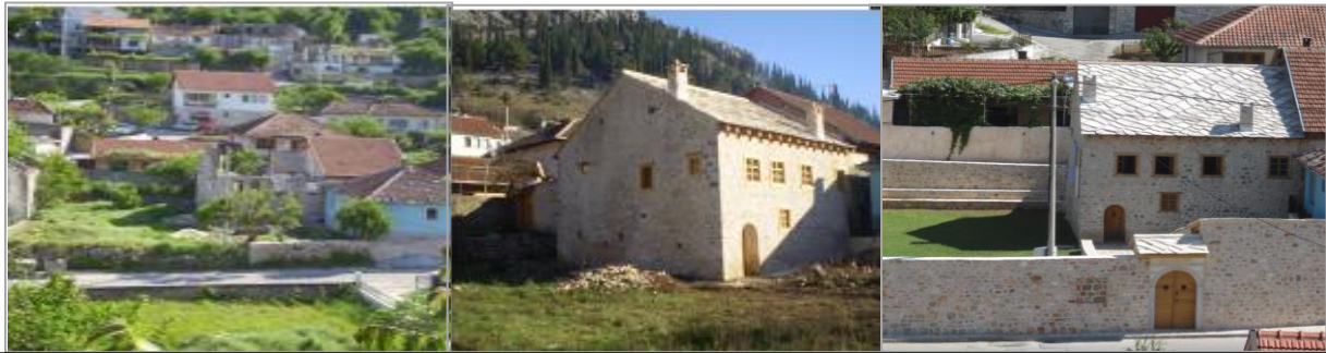
HIDR 1 before and after reconstruction
